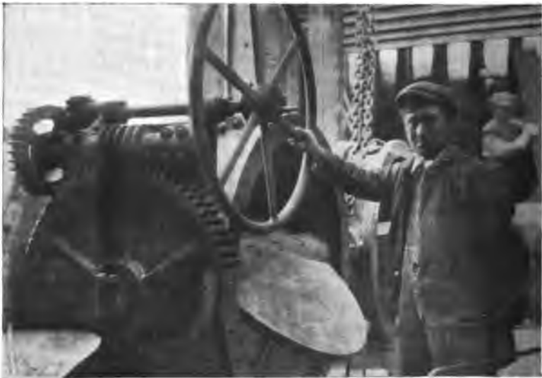
FIG. 174.—Butterfly Valve, Minitare Dam, Nebraska.
